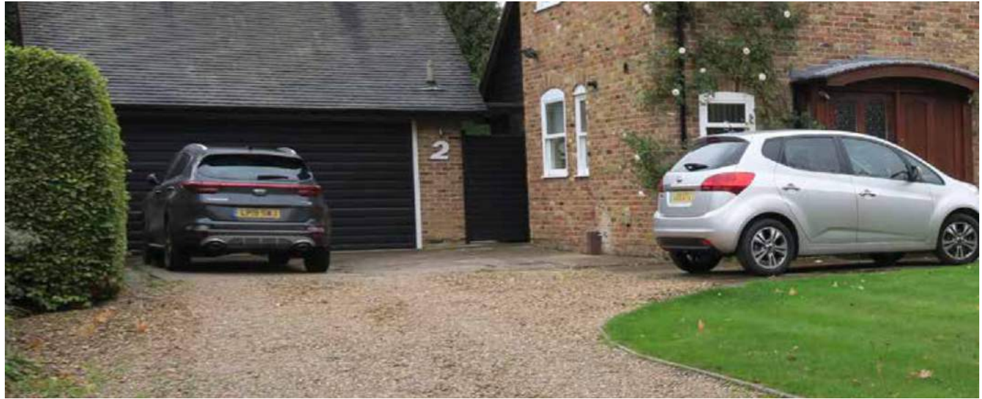
Figure 55: Side garage (left) designed as a secondary mass to the main residential building and built with a matching material palette.
