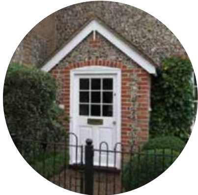
Flint and brick gabled porch
