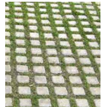
Figure 91: Permeable concrete paving.
