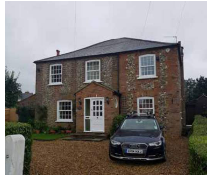
Figure 9: Building with red brick window trims and quoins and flint infilling.
