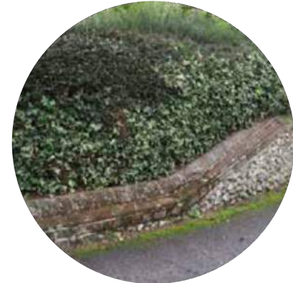
Low masonry wall with landscaped hedge
