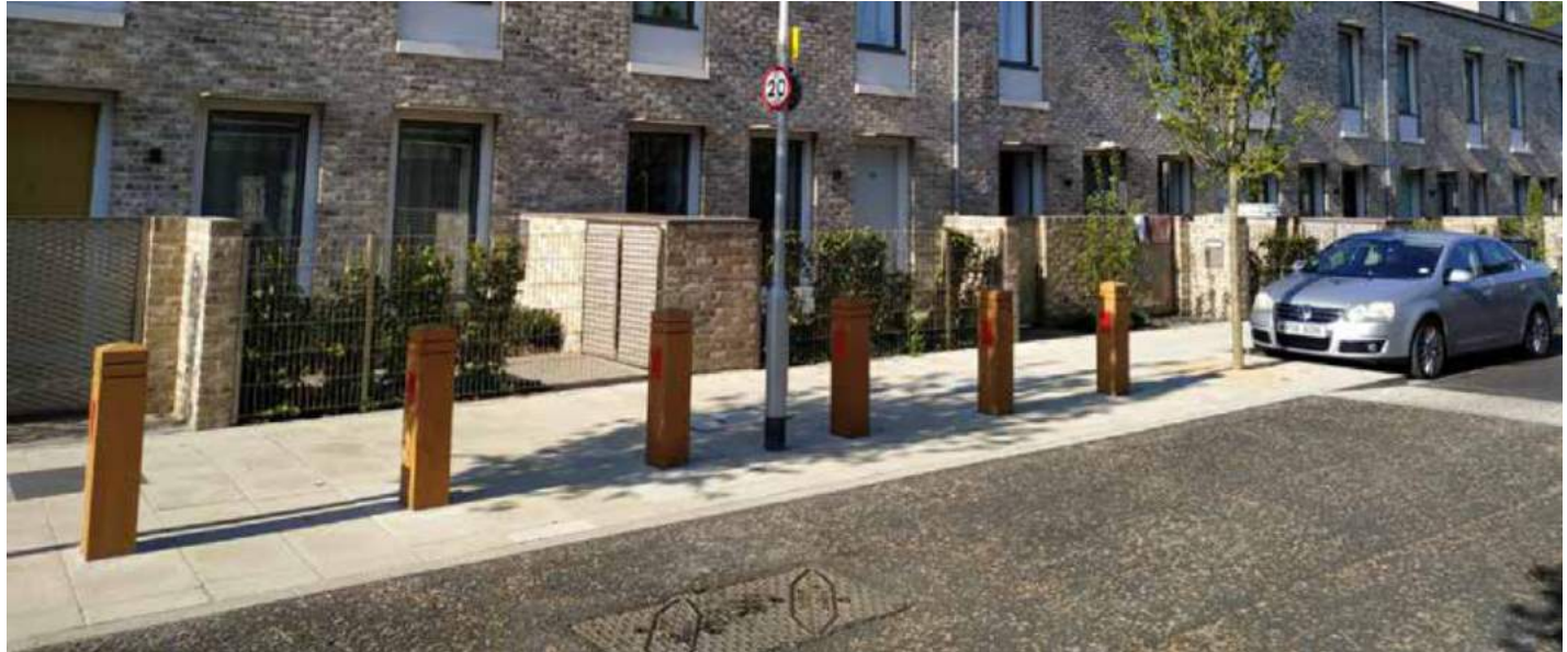
Figure 44: Example of a raised mid-block pedestrian crossing on a 20 mph street on Goldsmith Street, Norwich (note: many councils require blister tactile pavers at crossings to guide visually disabled pedestrians).
