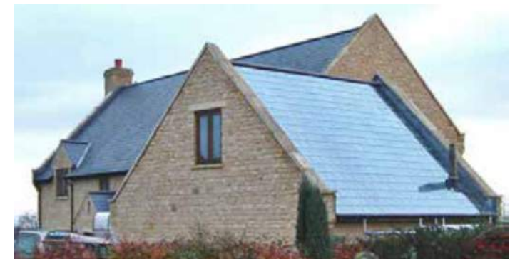
Figure 84: Integrated design for solar panels.
