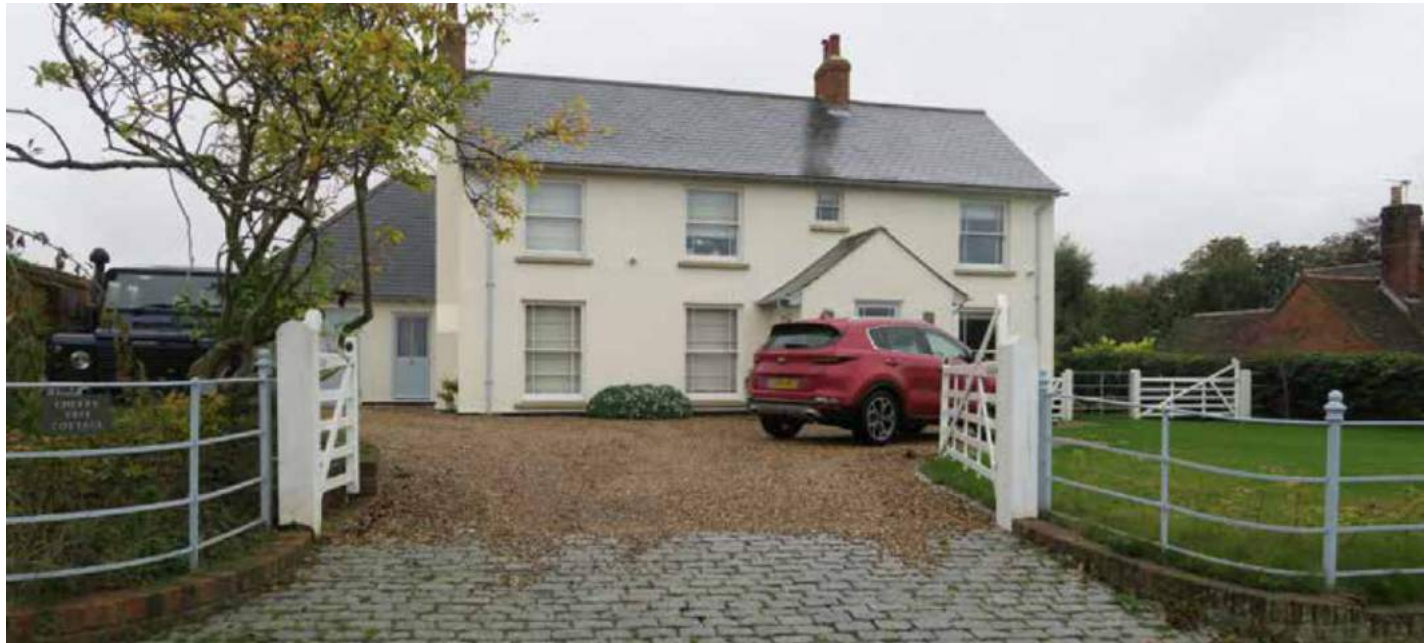
Figure 75: A recently renovated house along the Green, with consistent fenestration and a contemporary treatment of traditional materials.
