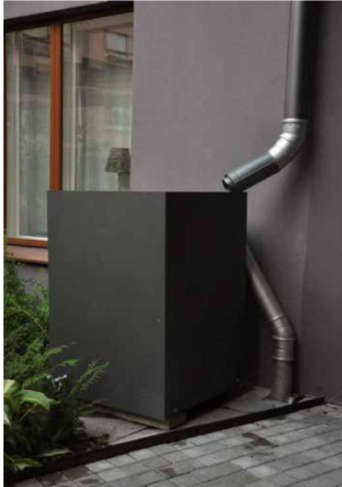
Figure 87: Examples of tanks used for rainwater harvesting.
