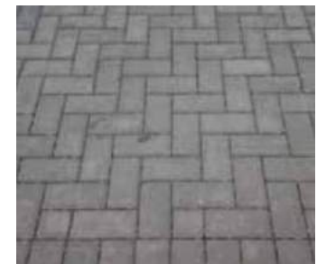
Dark grey concrete block paving
