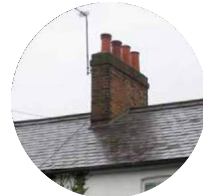
Red brick chimney
