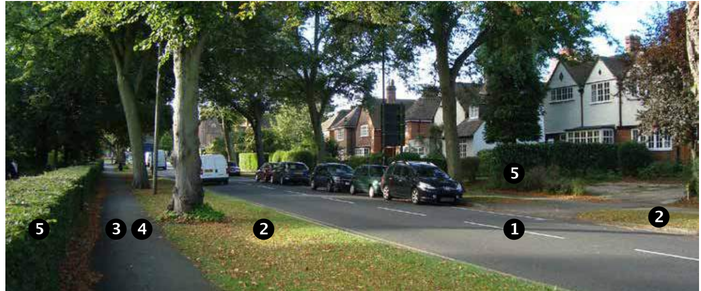
Figure 33: Primary road framed by wide tree verges in a residential neighbourhood. It is recommended that cycle provisions are separated from moving traffic and that parking bays, where required, are inset into the verges to avoid impeding the movement of pedestrians and vehicles.
