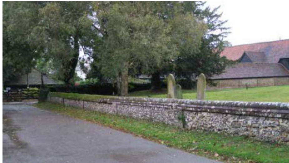
Figure 72: Church yard wall built with local flint.
