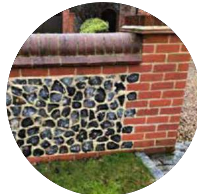
Knapped flint and red brick boundary wall
