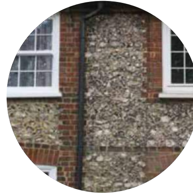
Red brick trim and knapped flint infilling
