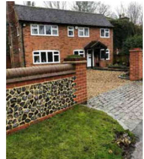
Figure 73: New wall using a mix of traditional local materials © Sarratt Parish Council.
