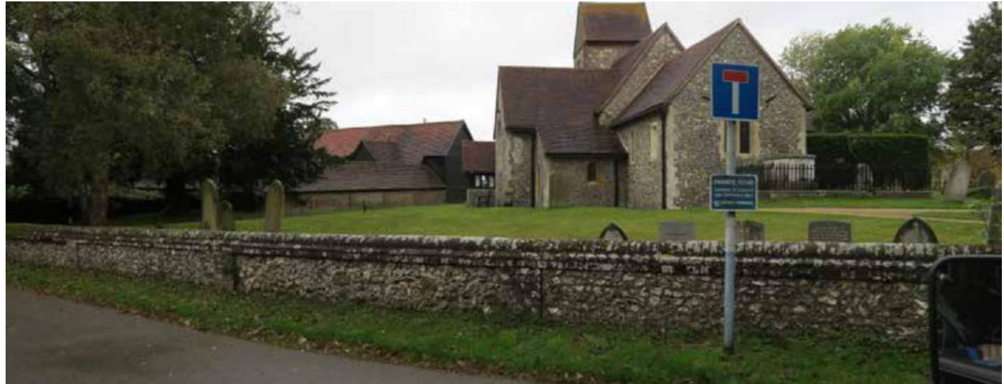
Figure 76: Flint boundary wall of Church of the Holy Cross.
